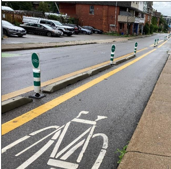
3. Locke Street, from Hunter to King * Note: the barriers depicted were added after the study period. The yellow markings are the original buffer-separated intervention.
