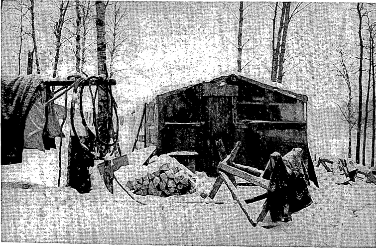
Photo. 2. An early winter camp, with a storage porch in front, and one room behind (approx. 3 metres by 6 metres) for the use of two families, Waswanipi, 1978. Winter camps vary in construction from wood frames with canvas or tar paper roofs (as here), to 'traditional' pole and canvas tepee-shaped lodges, to log cabins or one-room plywood dwellings. Excellent insulation is provided in mid-winter by banking snow up against the outside of the walls. The hoops on the right are to stretch and dry beaver skins.
