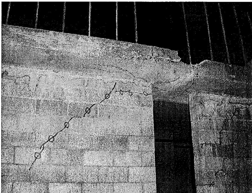
Figure 3.58: Cracking in Second Story of the South Portion of the Double Wall (Wall 2)
