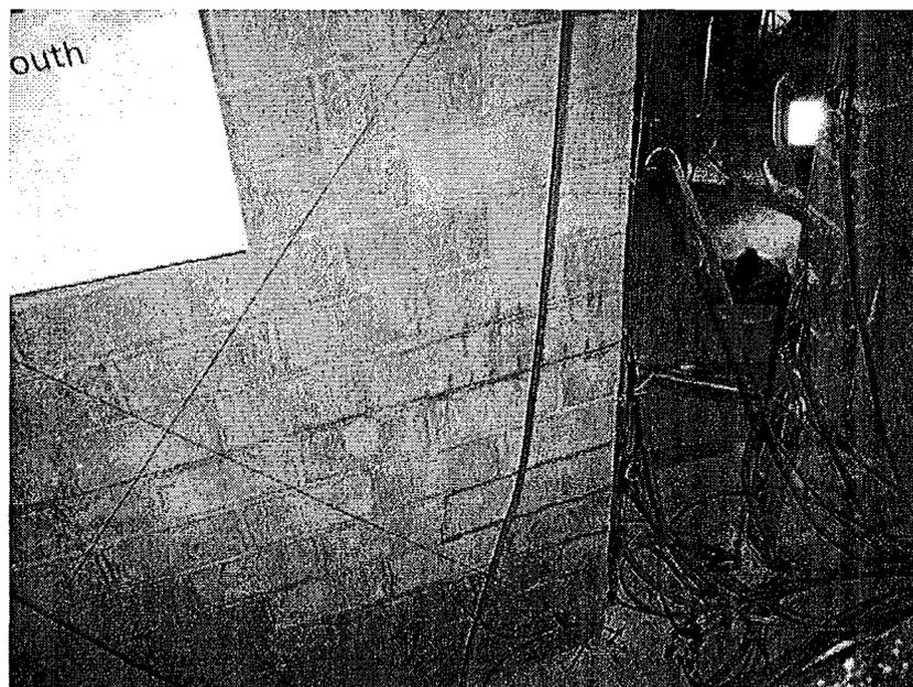
**Figure 3.20: Cracking on South Portion of the Double Wall (Wall 2)**
