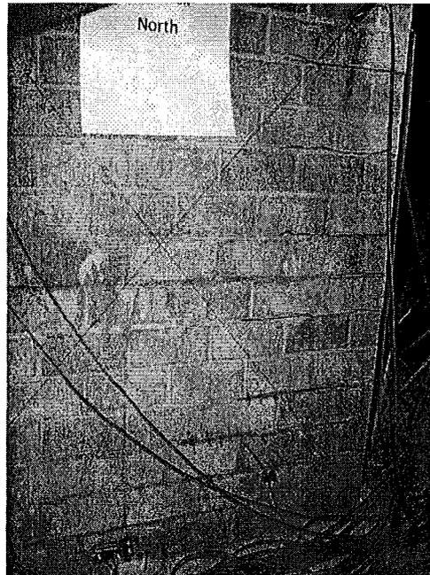
**Figure 3.19: Cracking on North Portion of the Double Wall (Wall 1)**
