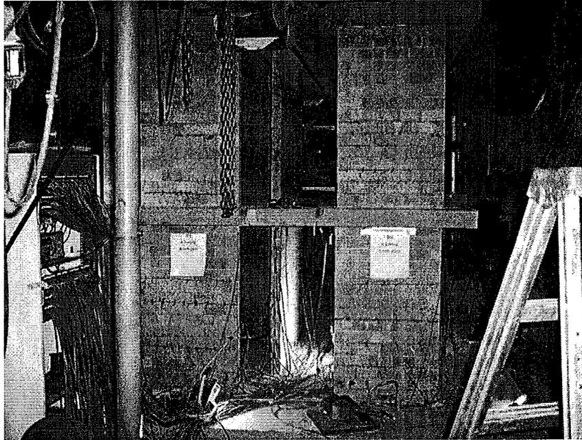
**Figure 3.35: Cracking on North East and North West Out-of-Plane (Walls 3 and 6)**
