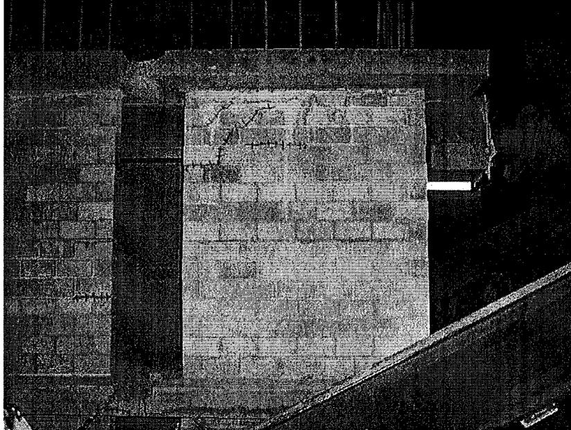
**Figure 3.32: Cracking in Second Story of the Double Wall (Walls 1 and 2) and First Floor Slab**
