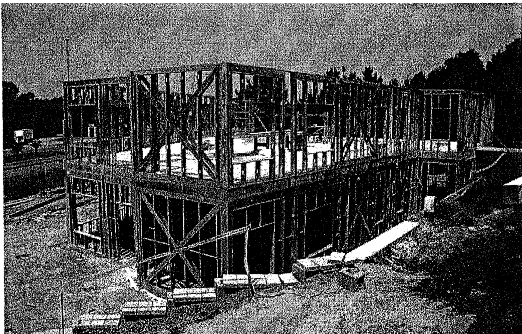
Figure 1.3 Two Story Commercial Building Framed Entirely with Load Bearing Cold-Formed Steel Members ( http://www.k2engineeringinc.com )
