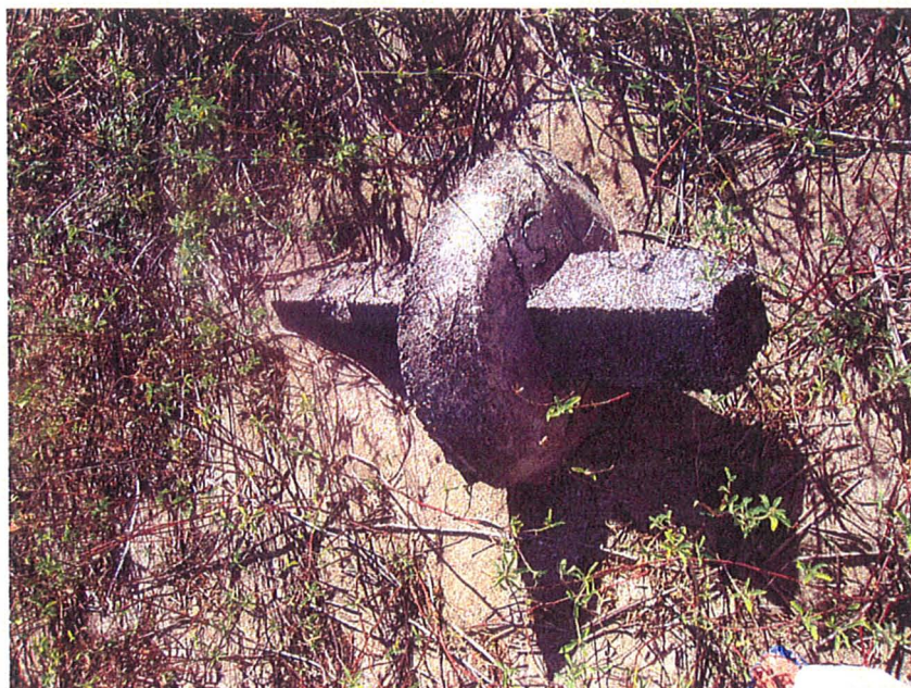
Figure 3.4: Example of the concrete markers located along the backshore of the beach that could not be used as a benchmark. The square 4"x4" post should be buried in the ground with the circular dish at ground level.
