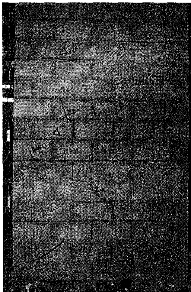
Figure 5-3: Wall 1 - Diagonal Tension Cracking at 2A_y yield
