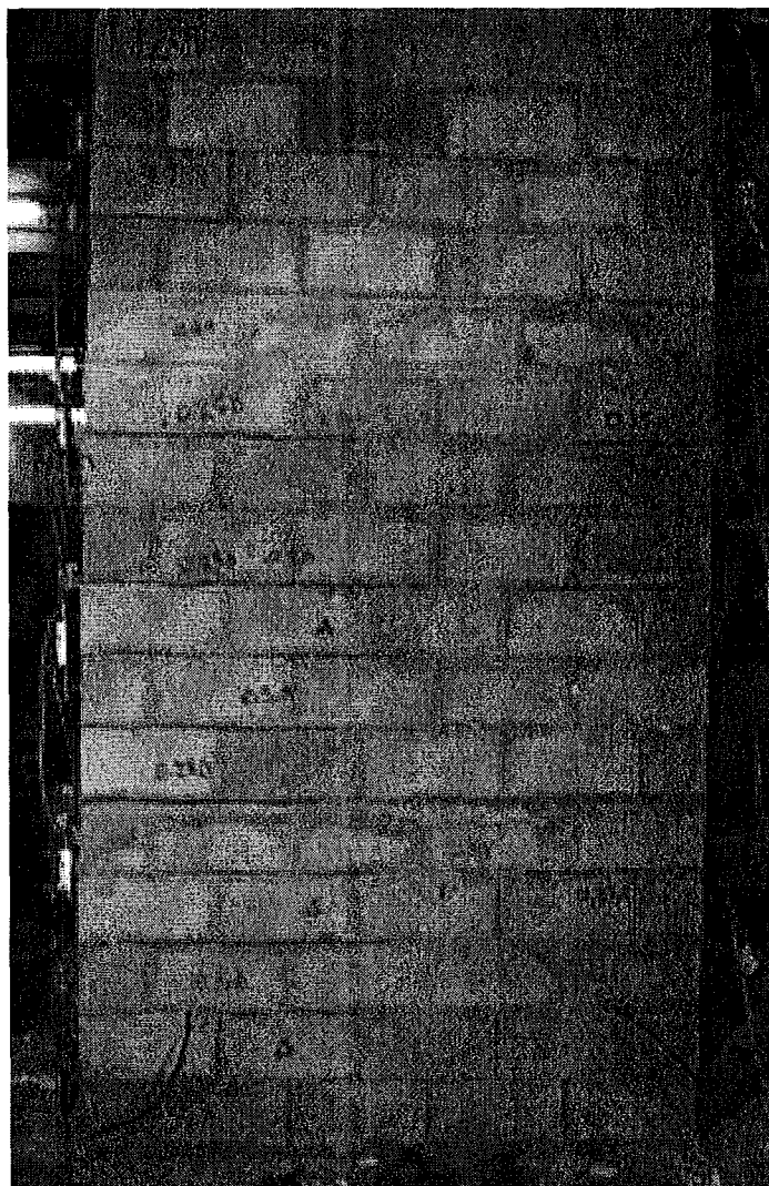
Figure 5-19: Wall 2 – Bed Joint Cracking at \Delta_y
