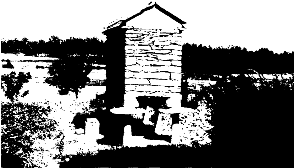
1. A granary built several decades ago with locally quarried granite (photograph by author, 1991).
