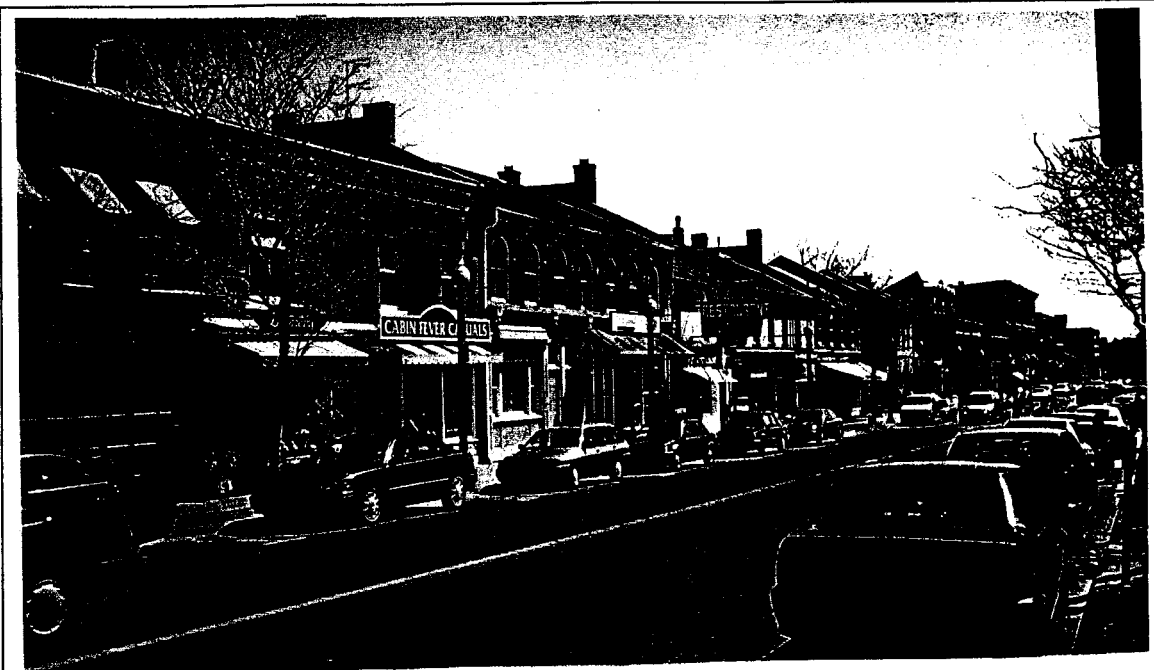
Figure 3.5: An example of the envisioned commercial streetscape from King Street, Dundas, Ontario
