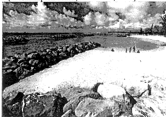
b) Beach protected by a system of detached breakwaters and a revetment (Sand Island, Ohio)
