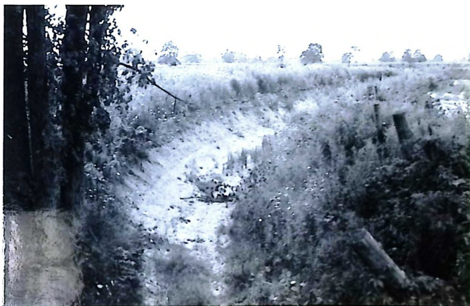
Illus. 8 North Forks Creek showing how natural drainage channels have been ditched and deepened to drain away excess water. This ditch was dry in late summer when the picture was taken.
