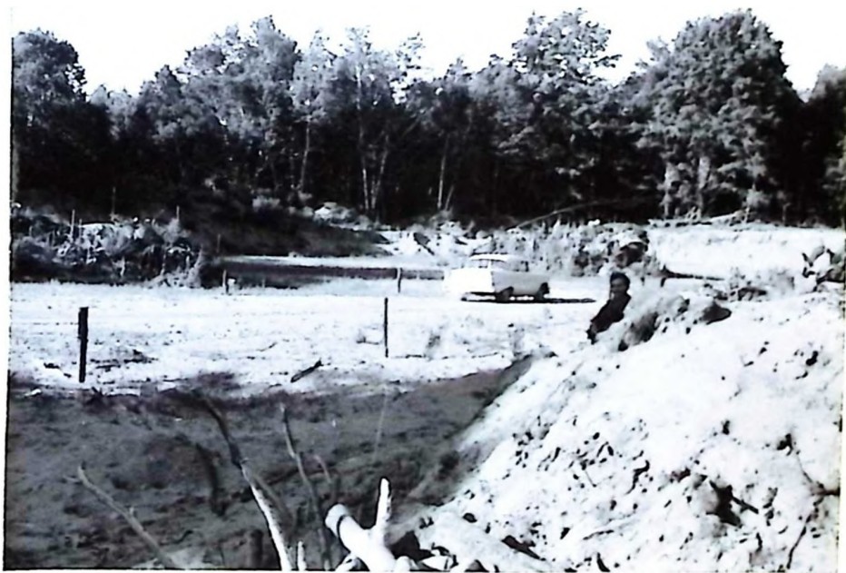
Illus. 19 A large sand pit in Woulton. Sand is excavated from sand hills to the level of the surrounding area. Township road runs right through the middle (between double fence). Side of pit is given by car. The material is used for road surfacing.
