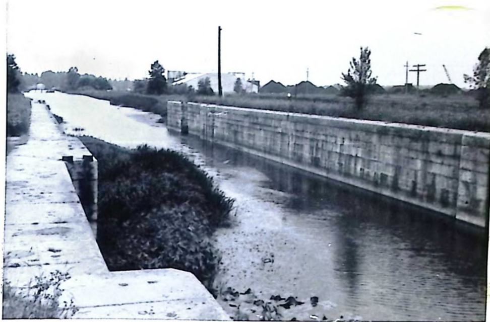
Illus. 16 Old canal lock at Port Maitland, showing solid stone construction and present condition of canal. In centre background is the new fertilizer plant being built and to the right of it the coal stock piles of the Canada Coal Co. beside the Grand River.
