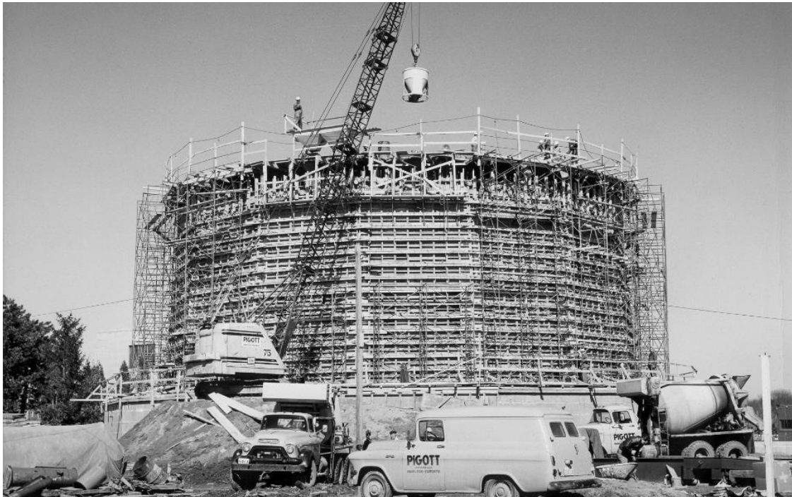
Figure 1: Image of the MNR being constructed, right before the concrete is poured. 8 They poured all of the concrete for the walls in one pour, taking 50 hours. 9
