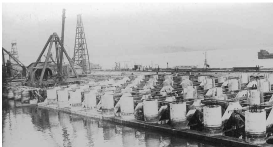
Fig. 8 Deck slab soffit falsework and formwork under construction, circa 1922, CVA 1376-315
