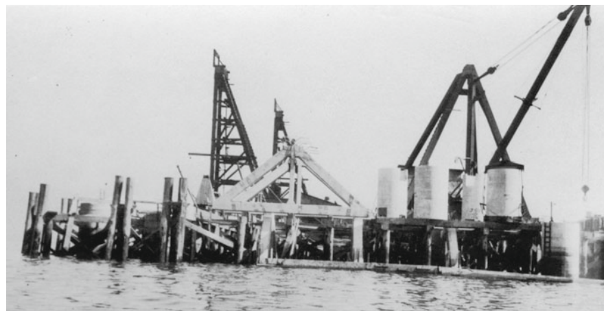
Fig. 7 Precast concrete sections and braces to be lowered into place, circa 1922, CVA 1376-314
