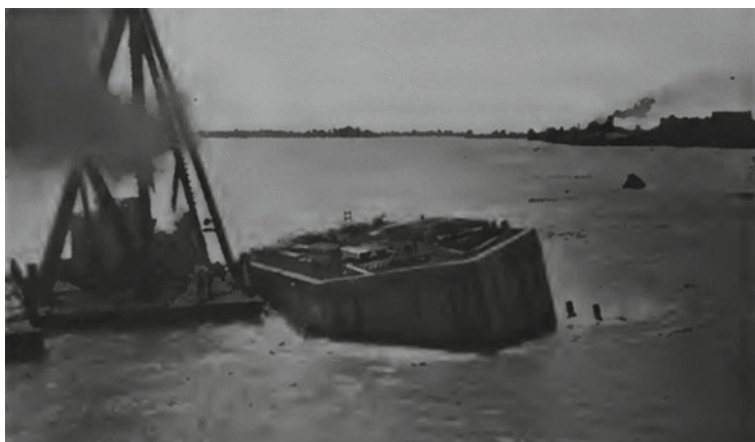
Fig. 6 Caisson 4 in distress. Source [2]
