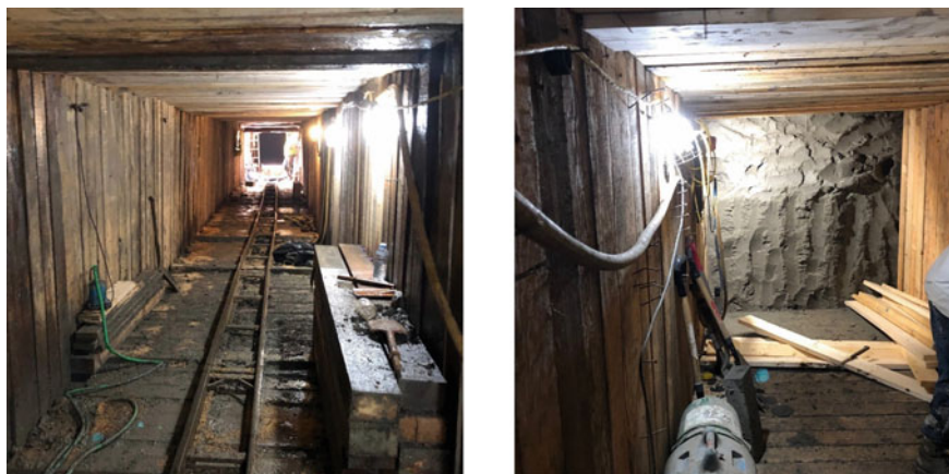
Fig. 9 Cap and lag tunnel under pearl street, shaft facing (left) and cut facing (right)
