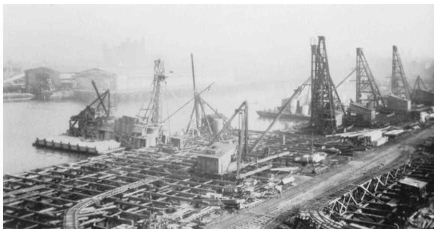
Fig. 9 Stiff-leg derricks to lift and rail tracks to transport materials on site, circa 1922, CVA 1376-316
