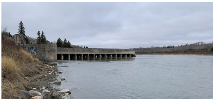
Fig. 6 Photograph of the dam at La Colle Falls in an oblique upstream view (taken November 2021). The navigation lock is located to the left, the incomplete dam in the center, and the open river to the right
