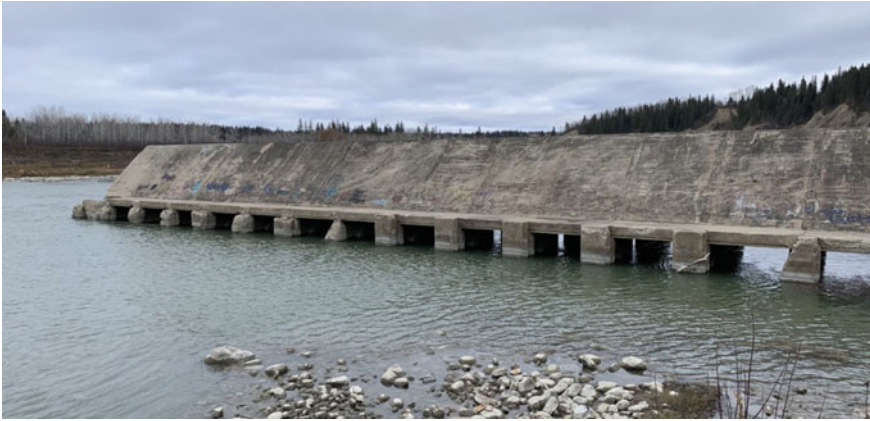
Fig. 4 Oblique view of the upstream side of the dam at La Colle Falls (taken November 2021). Note the outer end of the incomplete dam on the left side of the photograph and the throughflow port openings along the front face of the dam. The port openings had slots on either side so as to facilitate the insertion of stop logs once the dam was to be made operational
