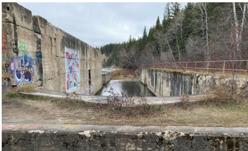
Fig. 5 Photograph of the lock at La Colle Falls viewing downstream (taken November 2021). The upper miter gate doors would close against the V-shaped concrete step in the foreground. The lock wall on the right was never brought up to full height. The guard rail located along this wall of the lock has simply been added as a safety precaution at the now-abandoned site
