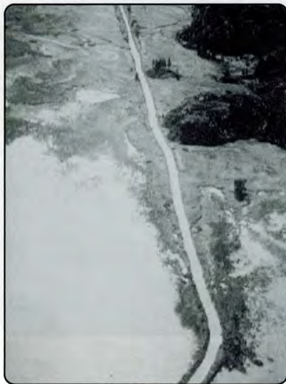
Photo 1. Aerial photo of Cootes Paradise in 1928, showing Desjardins Canal as it curved toward new outflow.
