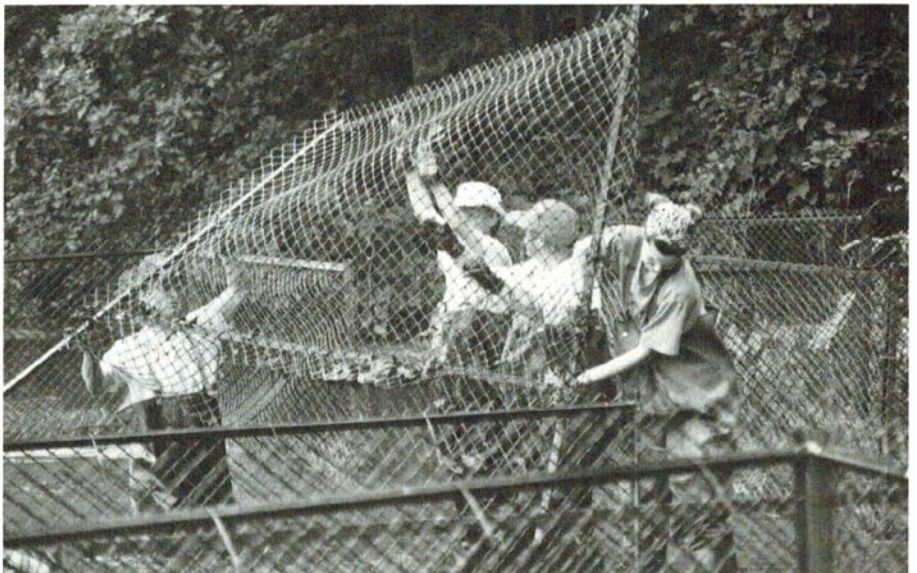
Eight-foot by eight-foot enclosures are built of four panels of weld-wire or plastic snowfence mounted with cable ties on T-bar frames. Volunteers construct the single panels on a board walk, and then carry them out into the marsh where the enclosures are assembled.
