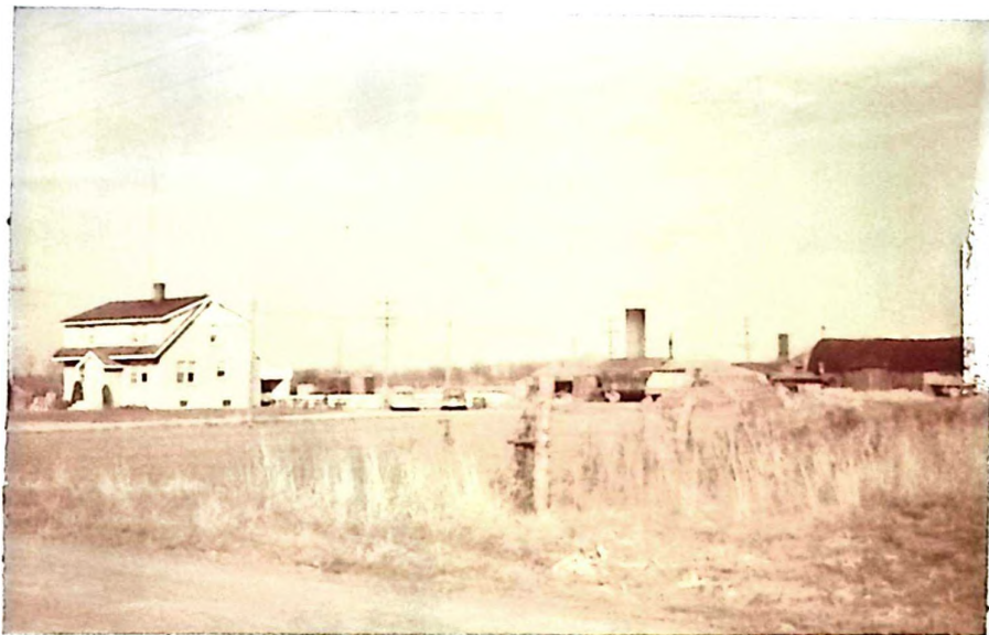
Photograph No. 37. Tile from Forest's tile plant is used to improve the field drainage on many of the local farms.
