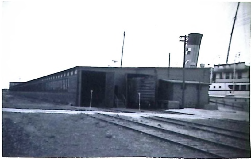
The C.P.R. package freight sheds at Port McNicoll.
