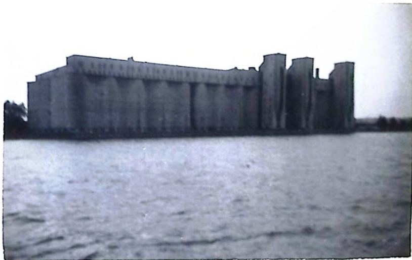
The grain elevator at Port McNicoll
