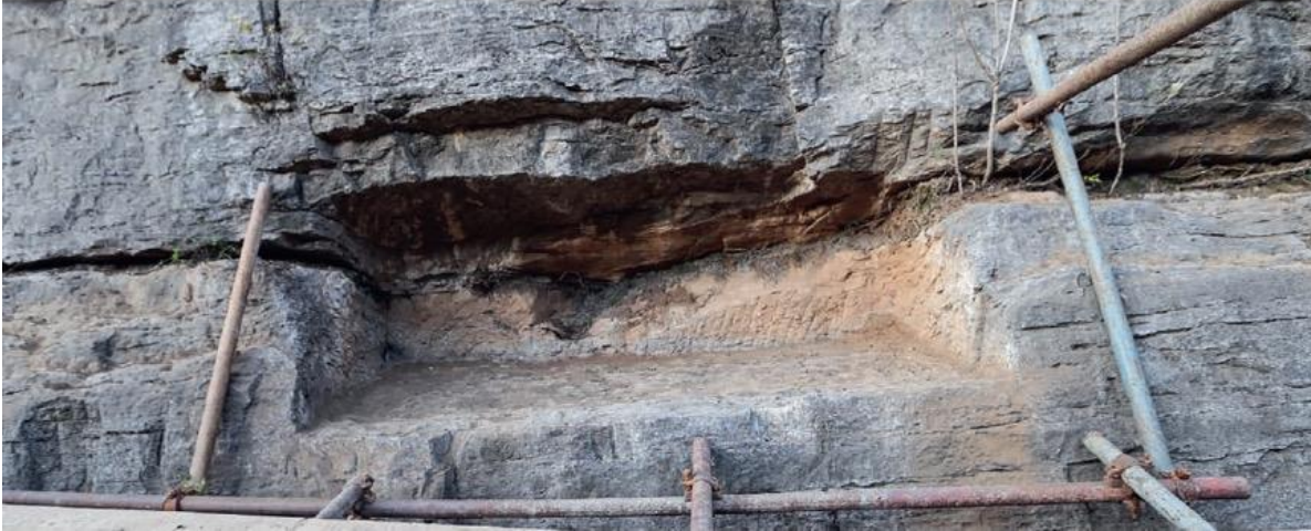
Fig. 3-32 WFG K2: Façade (Lan LI, 2016)
