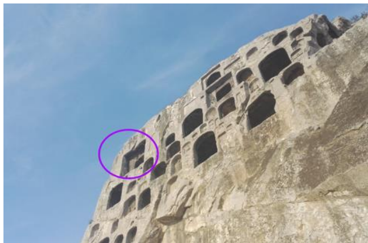
Fig. 5-16 Cave 964: Location (from below) (Lan LI, 2018)
