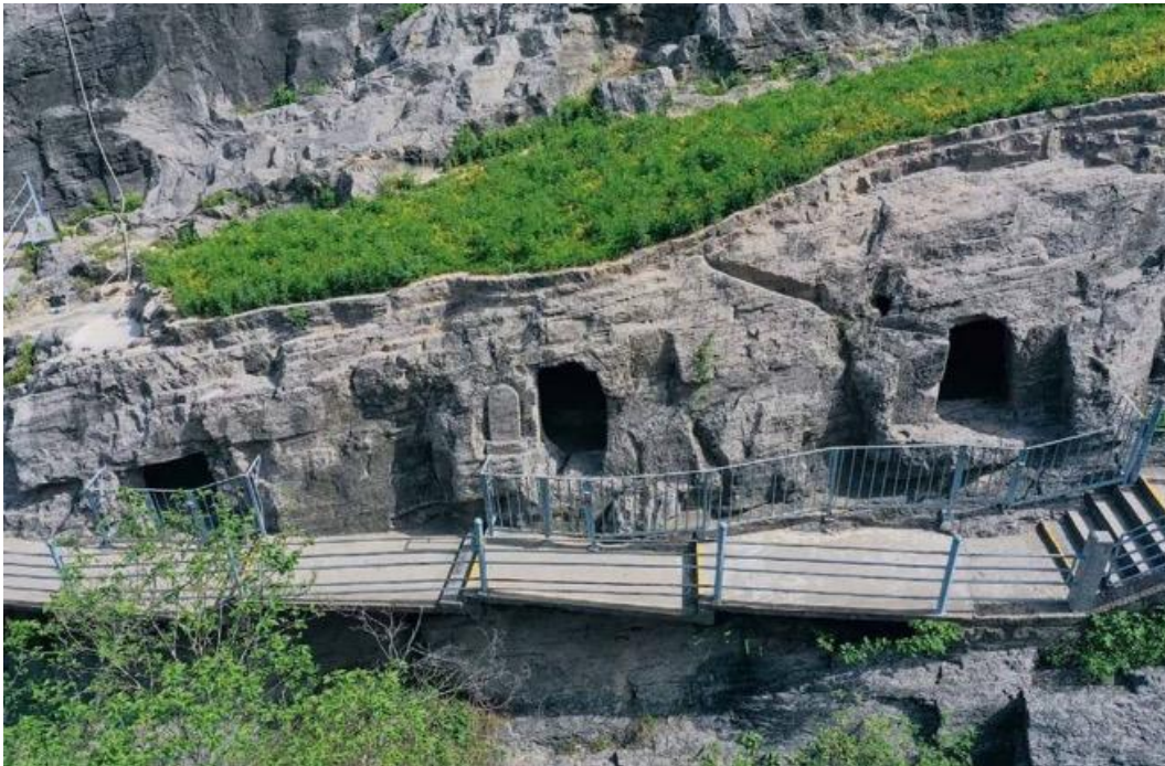
Fig. 3-18 An Aerial View of WFG K11-13, from Right to Left (LGRA, 2021)
