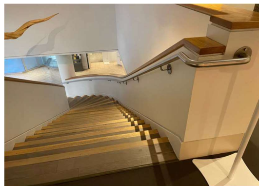
Figure 4.20 Nosings of the stairs at the Art Gallery of Nova Scotia
