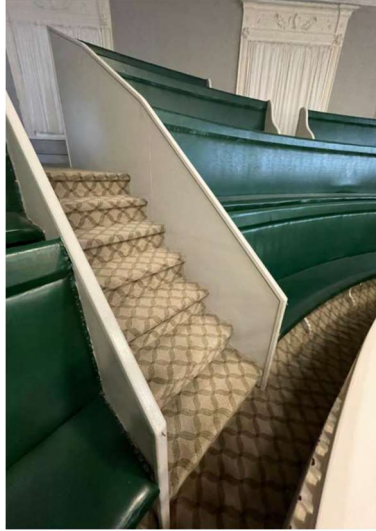
Figure 4.17 Steep steps in the gallery of Province House with inadequate handrails and narrow seats
