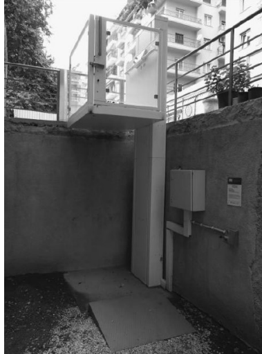
Figure 3.13 Lift installed in Acheiropoiitos, Greece [93]
