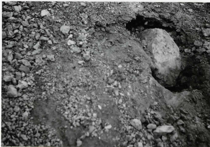
Figure 13.14 Excavation at site 14, Palliser Cone. This illustrates the mixture of fines and rock chips immediately below the surface of the upper and middle parts of this cone. Undisturbed surface material can be seen on the far left. The boulder is about 45 cm long. Compare with the site prior to excavation, sample 48, Figure 13.9A.
