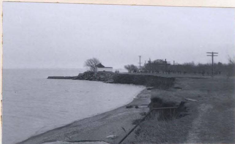
Fig. 32 A picture of the same section of the lake shore as above taken in March, 1953. The road has now completely disappeared as a result of the erosive action of the lake.
