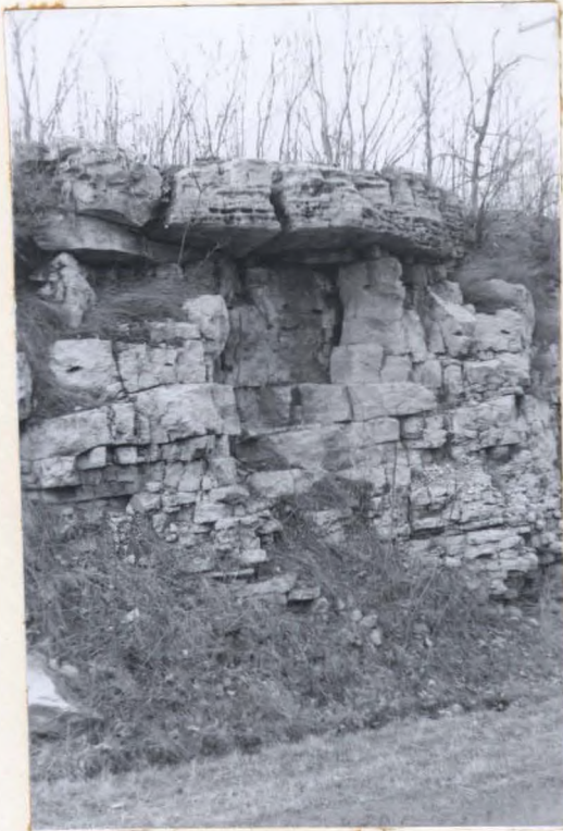
Fig. 1 An exposure of the bedrock along a road cut on the scarp-face south of Beamsville. The Lockport dolomite may be seen capping the Clinton formation.
