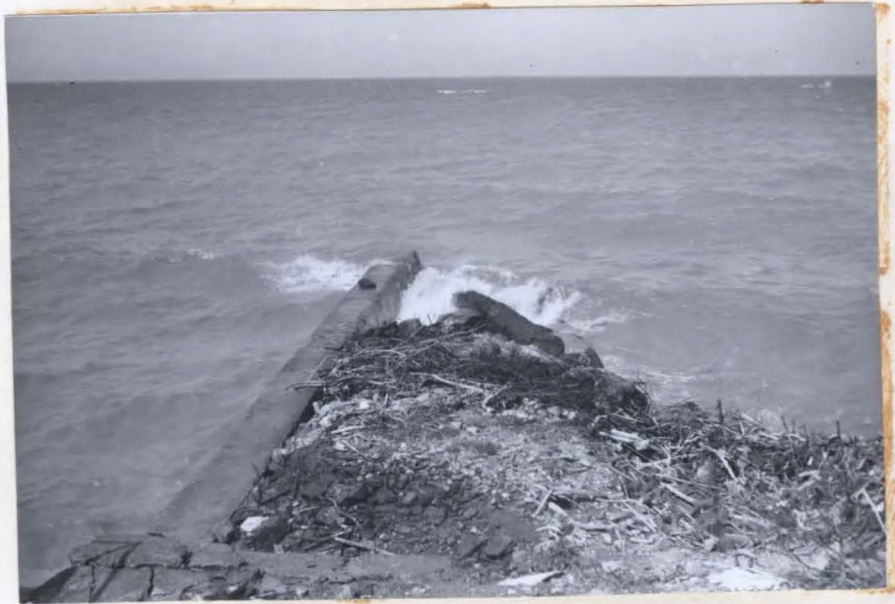
Fig. 35 A groin building up a beach along the lake shore. Very few of these exist in Clinton township.
