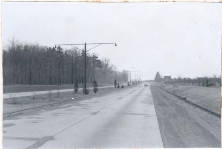
Fig. 10 A section of the Queen Elizabeth Way near Vineland.
