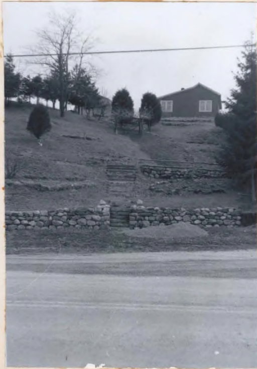
Fig. 25 A house situated on top of the Iro- quois shore-cliff east of Beamsville. Highway No. 8 is visible in the fore- ground.
