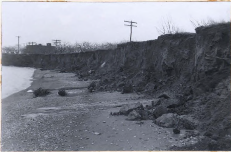
Fig. 33 An example of slumping along the Lake Ontario shore-cliff.
