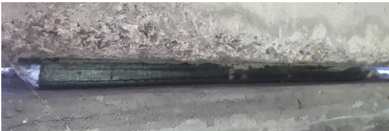
Figure 18: Undamaged bearing at German Mills Creek; no liquid visible
