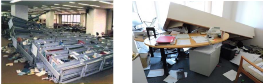
Fig. 1-1. Overturned nonstructural components [10, 11].
