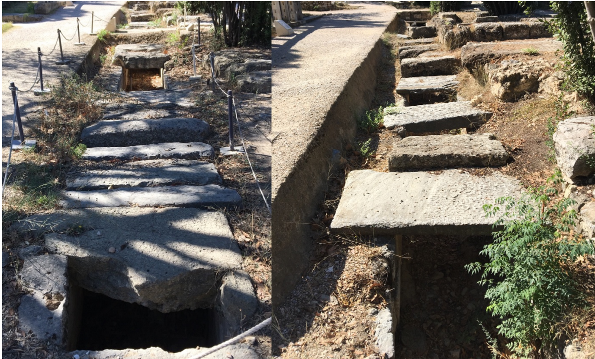
Figure 8c and 8d. Photos by the author of a Great Drain channel showing the interior and roof slabs.
