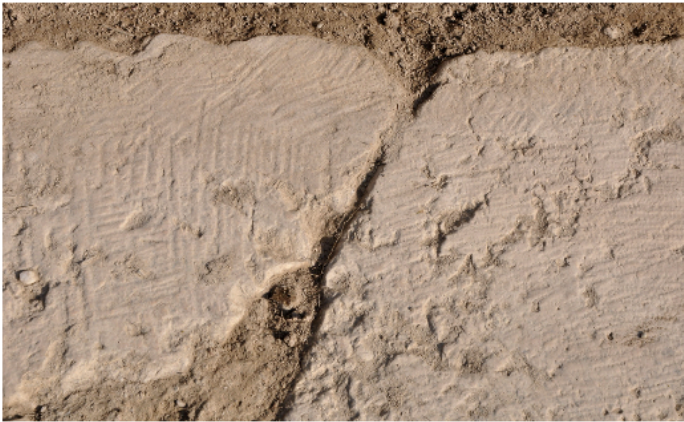
Figure 6a. Northeast corner of the Southeast Fountain House with claw-tooth chisel marks visible. Sourced from Paga, 2015: 365.
