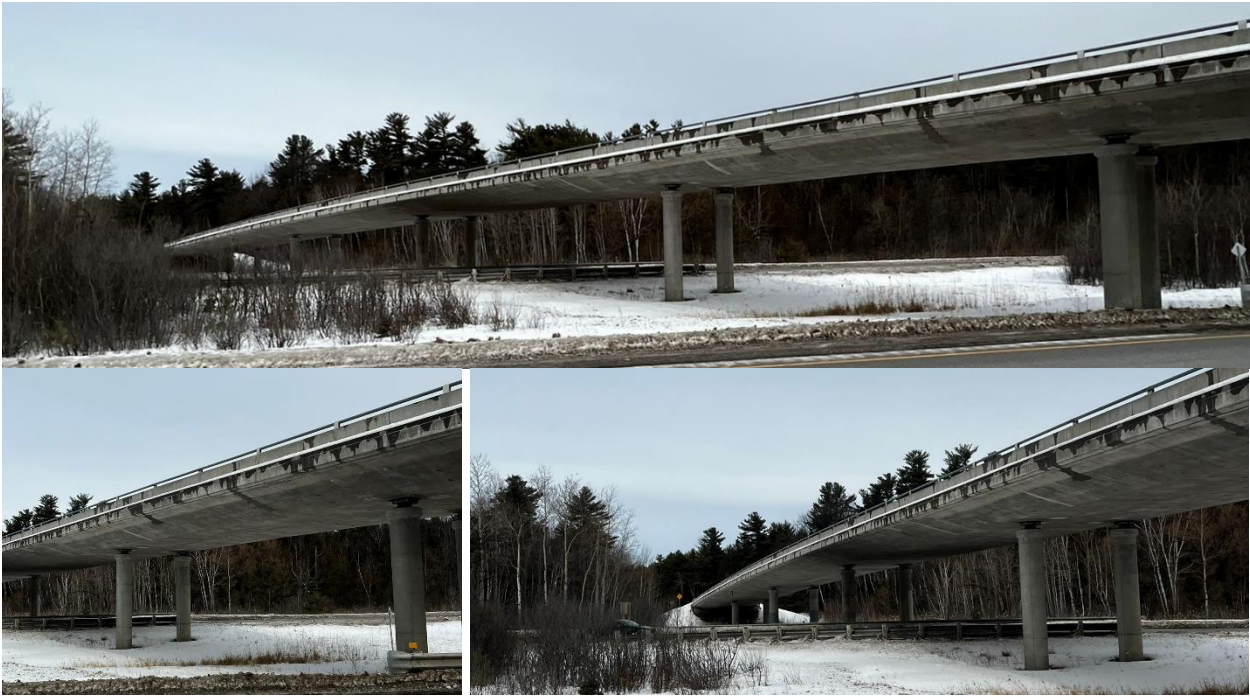
Figure 2.2. The overpass over the highway
