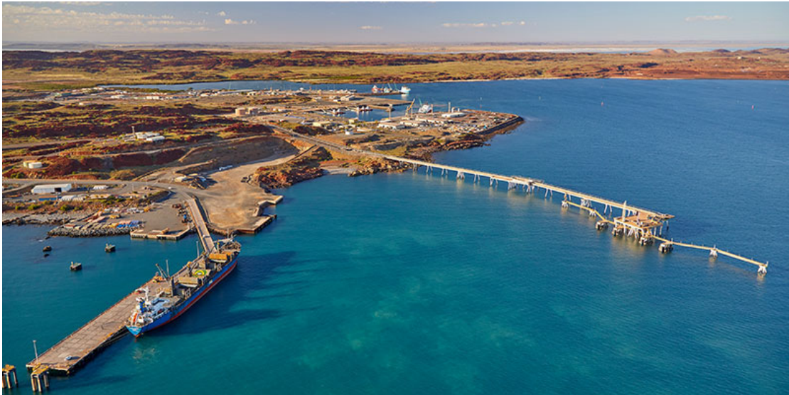
Figure 1. Cargo wharf (left) and LNG jetty (right). (Port of Dampier, Pilbara Ports Authority, Australia, n.d.)
