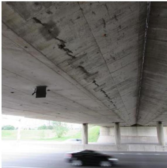
**Fig. 2.2** A bridge with a BCI approaching 70: Deck soffit with wet longitudinal cracks and delamination
