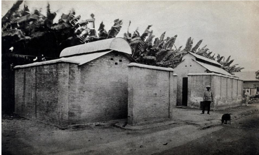
Figure 3.6: Lagos latrine buildings, 1910
