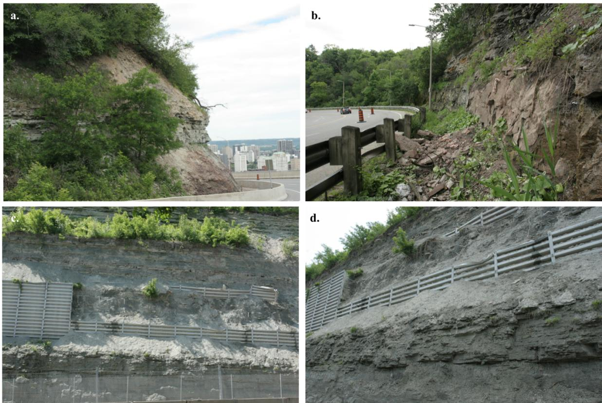
**Figure 3:** Access roadways cutting through the Niagara Escarpment in Hamilton and associated erosion of steep marginal slopes (a) top of the Jolley Cut roadway and view of lower downtown core, (b) small bedrock slide along the Jolley Cut, (c,d) failed infrastructure installed to prevent erosion along the Sherman Cut roadway (Lee, 2018).
