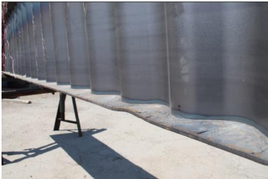
Figure A-6: Local Flange Buckling of the Deformed WTA500/127x6
