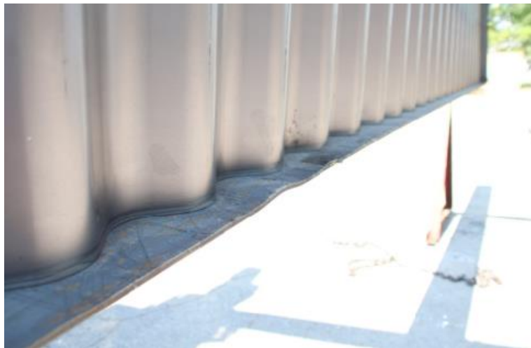
Figure A-9: Local Flange Buckling of the Deformed WTA610/127x6
