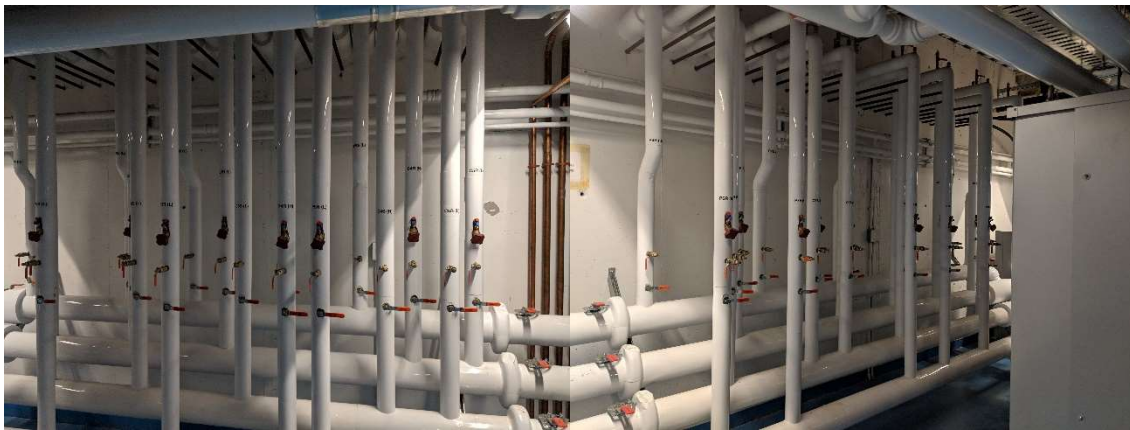
Figure 3.2 - Borehole String Connection to Header
