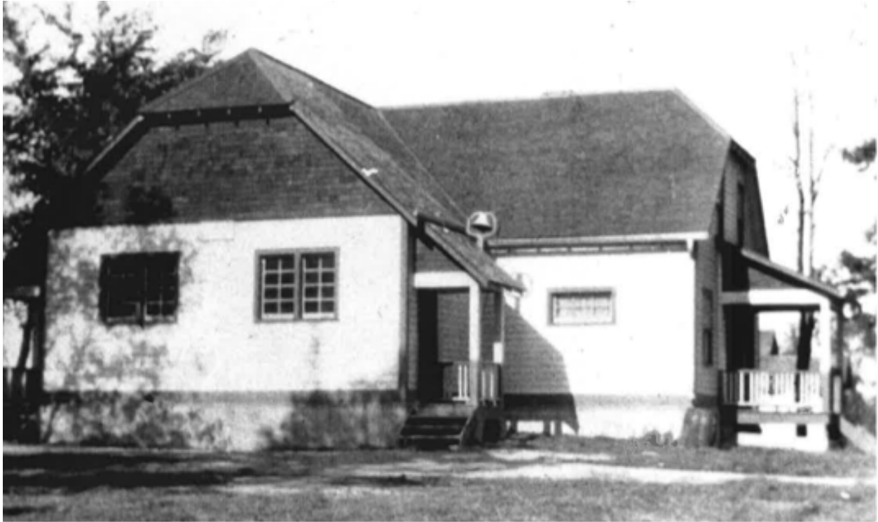
No. 6 School. Built sometime between 1878 and 1903 and located at the intersection of Fourth Line and Cayuga Roads. The school was known colloquially as 'the pumpkin' because of its rounded roof. As a student, 6Ned remembered a friend stuffing newspapers into the floorboards to keep the snow from coming into the school. Courtesy of Oliver M. Smith-Kawenni:io Elementary School.
