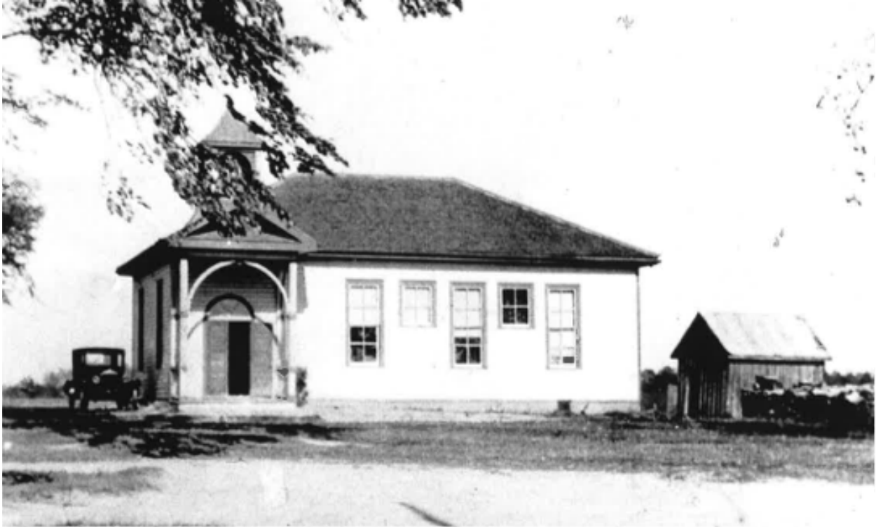
No. 3 School. Built in 1912 and located at the intersection of First Line and Mohawk Roads. Ed became teacher-administrator of the three-room schoolhouse in 1966 and later full-time principal into the 1980s. It is the school where Ed found exposed asbestos after examining an exterior loose board during one of his yard duties. My father attended the school as a child in the 1970s. Courtesy of Oliver M. Smith-Kawenni:io Elementary School.
