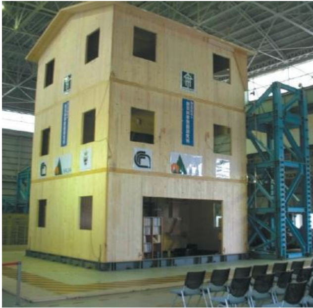
(a) Three-storey CLT house tested at NIED Laboratory, Japan [Gagnon and Pirvu, 2011]
