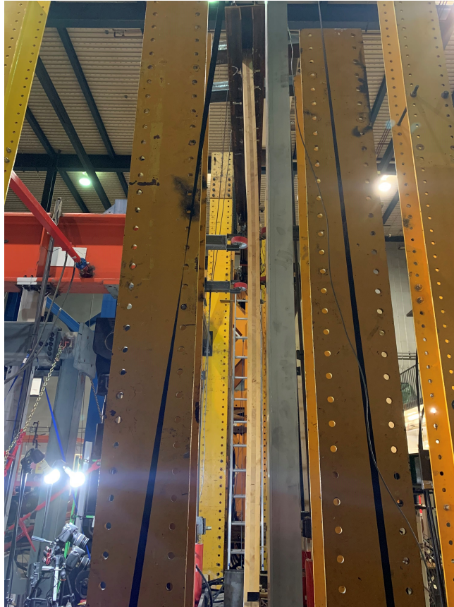
Figure 5.12: Out-of-Plane Buckling Wall Failure
