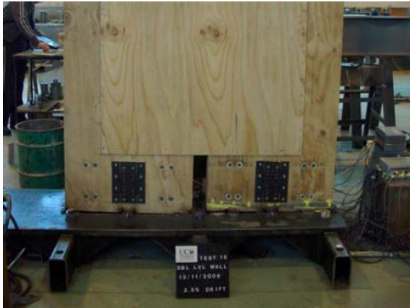
Figure 2.8: Plywood Coupled Wall-to-Foundation Test from [Smith et al., 2007]
