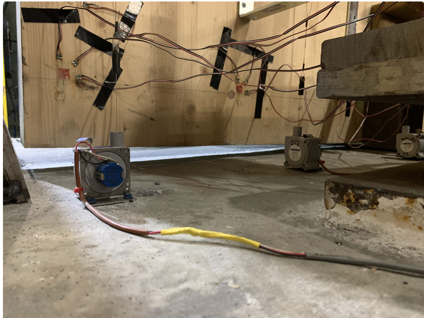
Figure 5.11: Decompression Toe at 3.0% Drift
