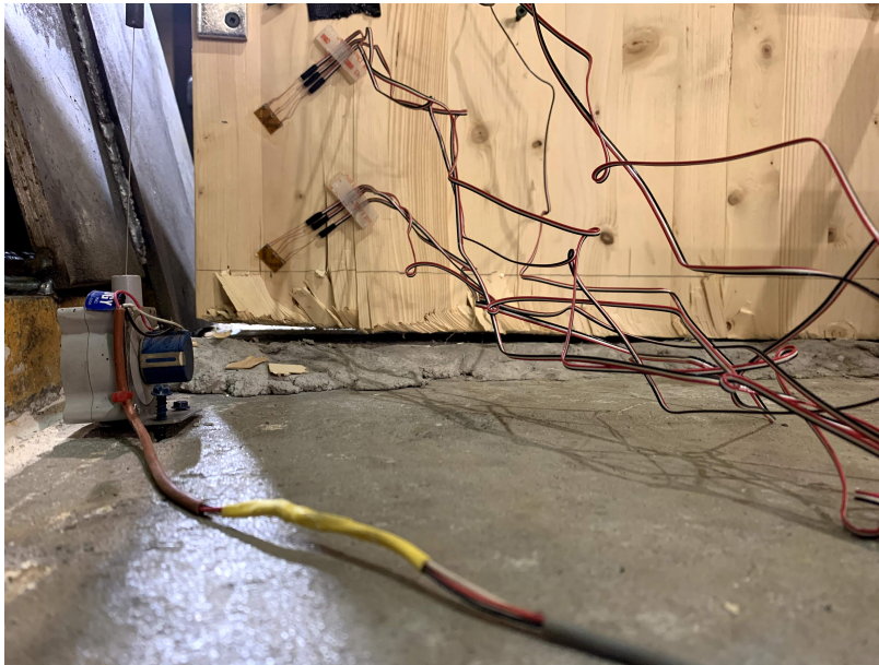
Figure 5.5: Permanent Damage to Rocking Toe after 3.0% Drift Cycle
