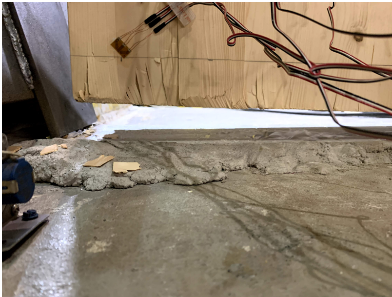
Figure 5.4: Decompression Toe at 2% Drift
