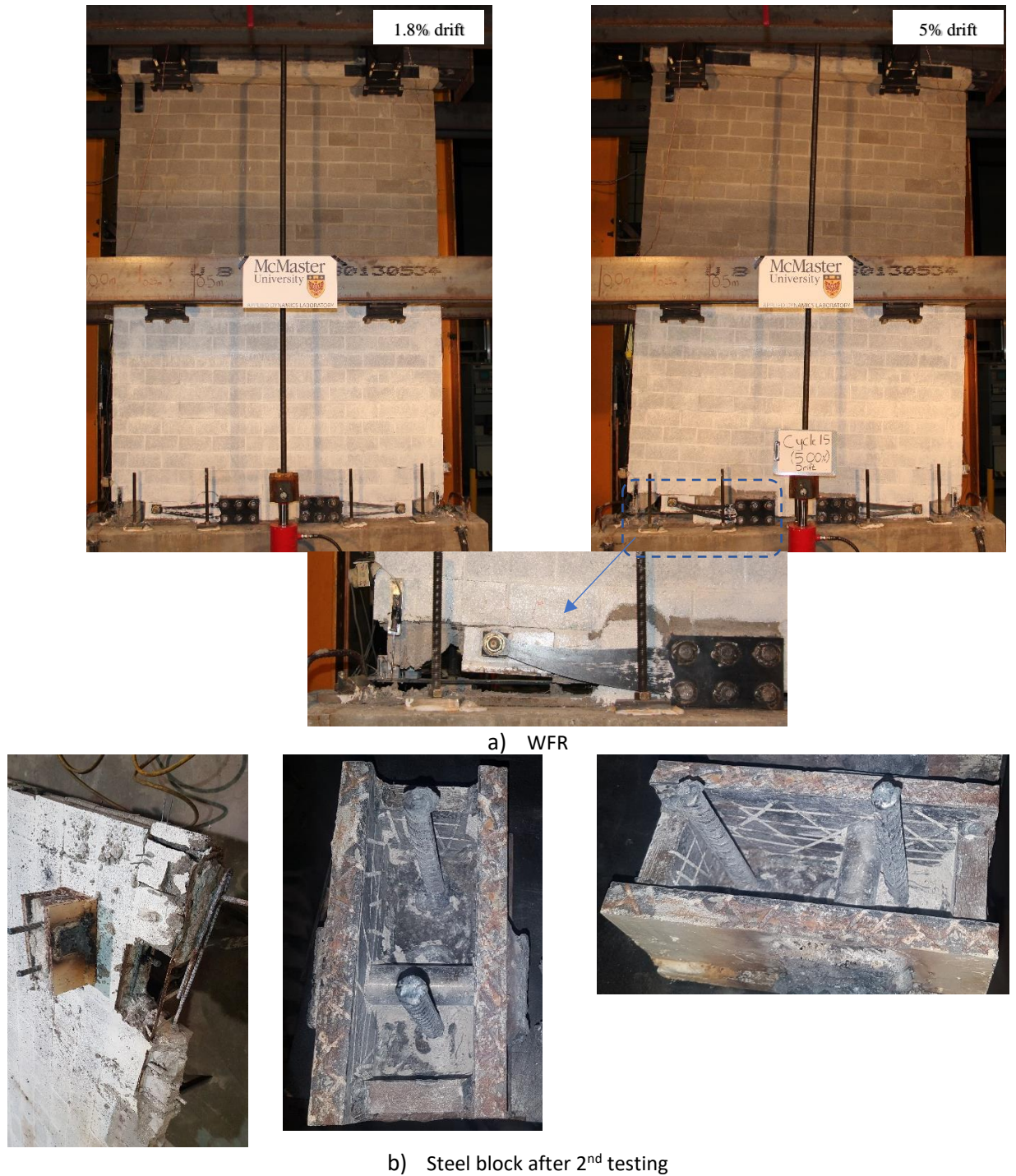
Fig. 5.9. a) Damage of wall WFR, b) Steel block condition after testing wall WFR
