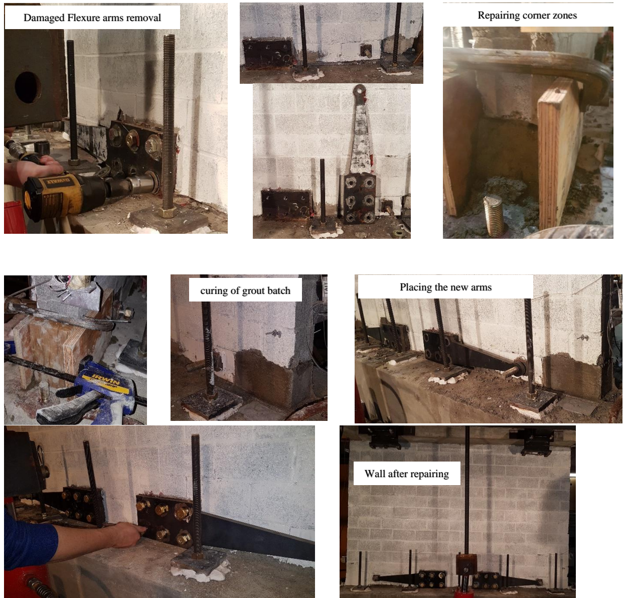
Fig. 5.8. Repairing stages of wall WF
