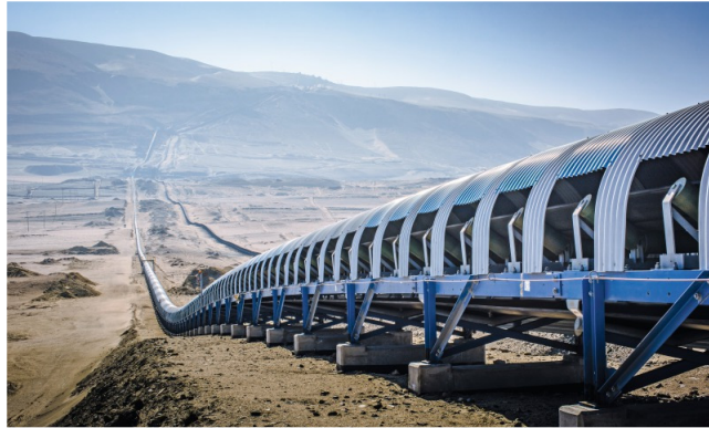
Fig. 1.2 Downhill Conveyor System [1].
