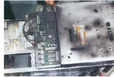
(f) Dust Accumulation into Drive Enclosure
