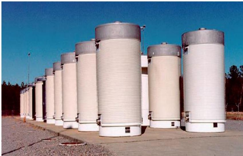
**Fig. 2.9** Arranged CASTOR V/21 vertical casks at Surry Nuclear Power Station, Virginia, USA, (Skrzyppek and Kim, 2015)
