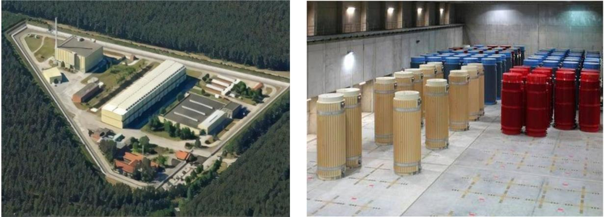
**Fig. 2.10** A site view for Gorleben interim dry storage facility (on the left) and an interior view that shows arranged vertical CASTOR casks stored indoors in the same facility (on the right) (Fraczek, 2013)
