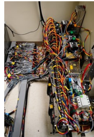
(b) Phase-shifting Transformer
