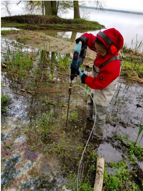
Figure 4.2. Photograph of Tammy Hua demonstrating the use of a hammer drill to install a mini-profiler into the subsurface (not HB site). Tubing is pumping water into the ground to prevent clogging of ports.
