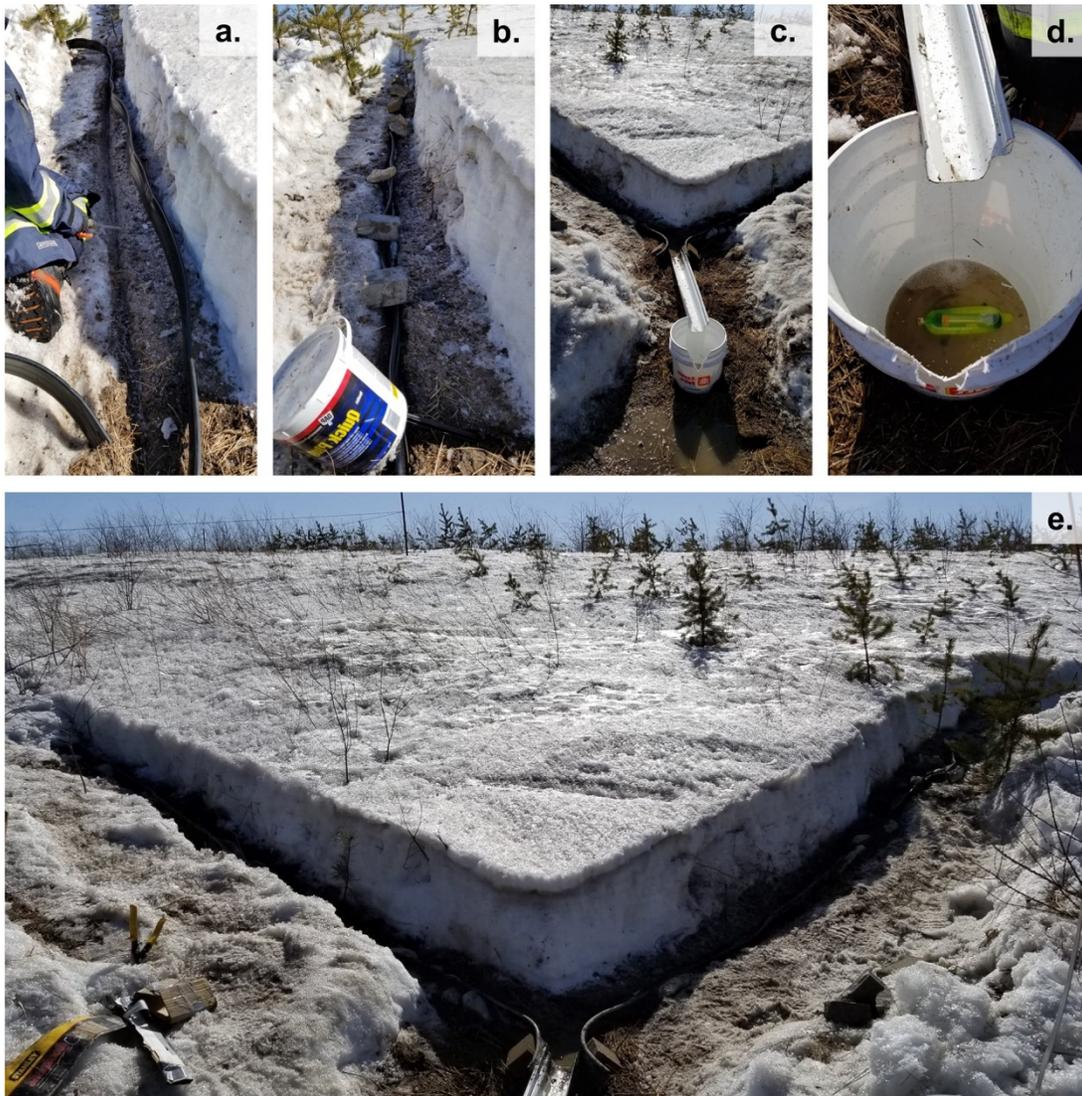
Figure 3.2. Runoff collector construction phases. a) Two 10-15 cm trenches were dug into the frozen ground, b) hydraulic cement was used to seal the garden edging into the trenches, c) trenches tapered at the bottom of the slope to form a “V” where an eavestrough was used to funnel water towards the bucket with a v-notch, d) a pressure transducer was used to continuously measure water height and discharge, e) completed runoff collector where each arm of the “V” was ~4 m.
