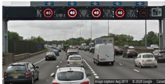
Fig. 1.1. VSL signs on the M25 highway in the UK (Map data © 2020 Google)
