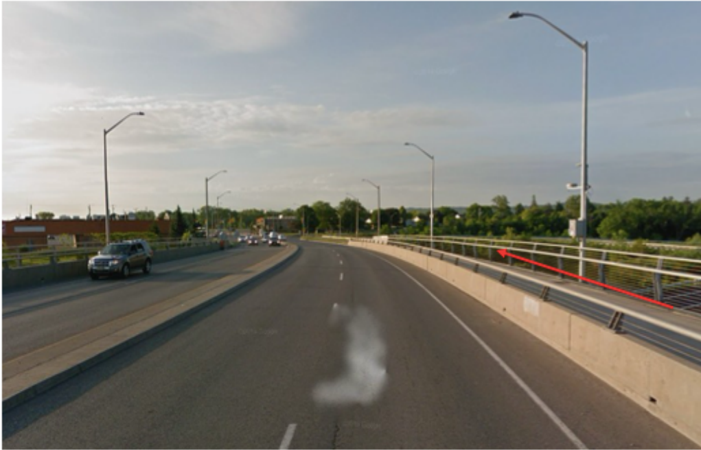
Figure 20. Segment 30 of route 2B depicting the protected multi-use trail on the right side of the roadway on an arterial road over the Red Hill Valley Parkway (Source: Google Street View).
