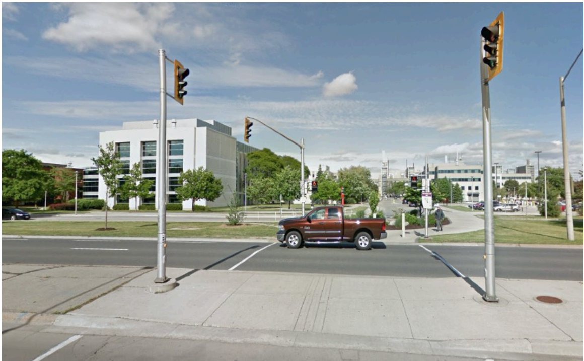
Figure 8. Segment 13 of route 1A depicting a pedestrian-activated signal to cross a an arterial road (Source: Google Street View).
