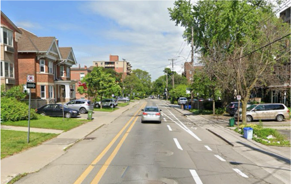
Figure 29. Segment 4 on route 3B with a buffered on-street bicycle lane on a one-way street (Source: Google Street View).
