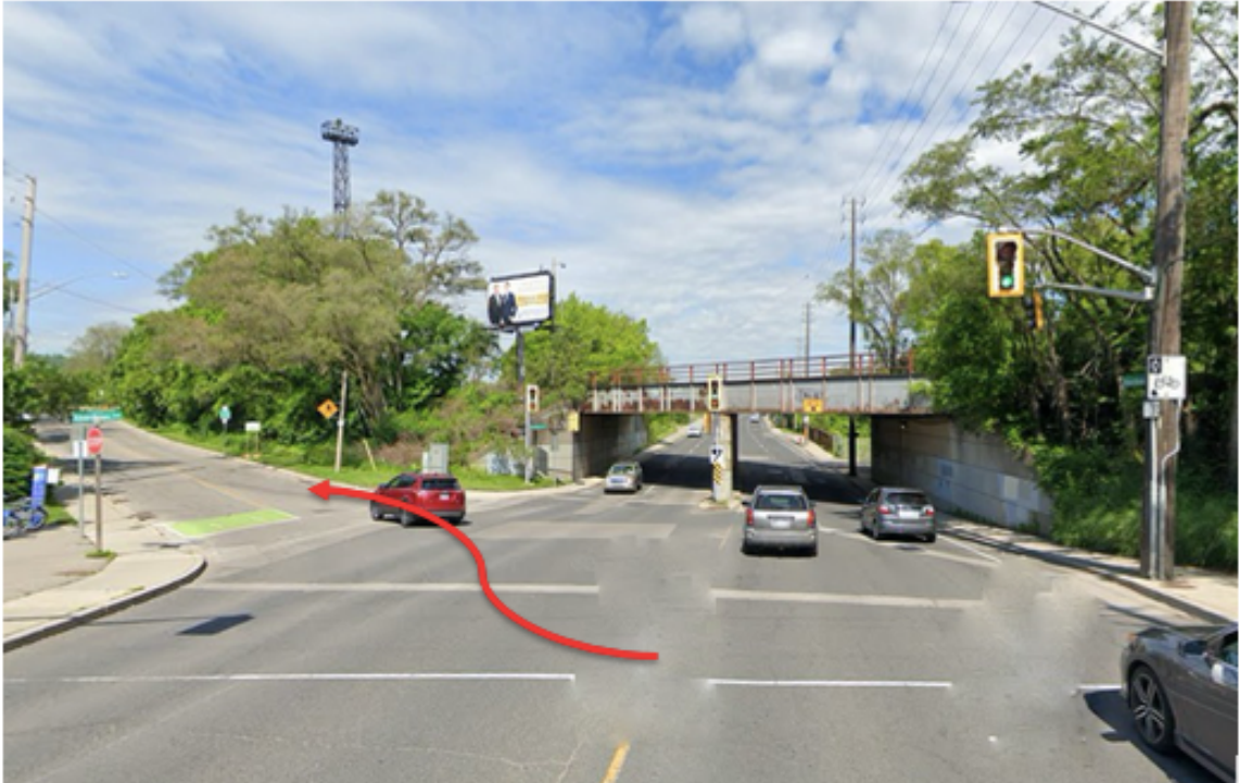
Figure 16. Segment 14 of route 2A depicting a signalized intersection where a cyclist would turn left on to a street with sharrows to travel to the Hamilton-Brantford Rail Trail (Source: Google Street View).
