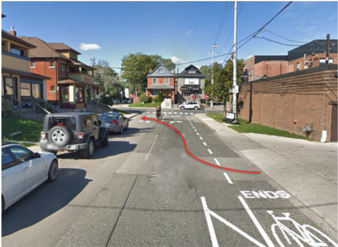
Figure 14. Segment 8 of route 2A depicting the buffered bicycle lane ending and the transition that a cyclist would have to make to get into the left-turn lane (Source: Google Street View).
