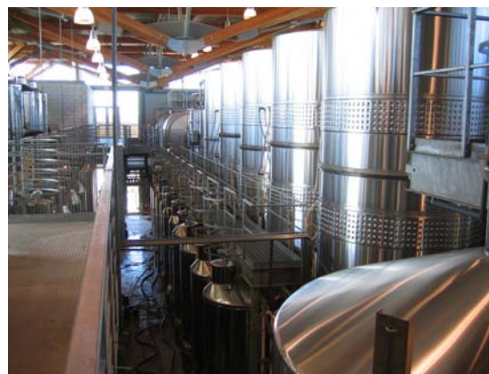
FIGURE 9: FERMENTATION ROOM. Several temperature-controlled stainless-steel tanks, some of capacities up to 25,000 L in Jackson-Triggs Winery in Niagara-on-the-Lake, Ontario (Eriksson, 2006).
