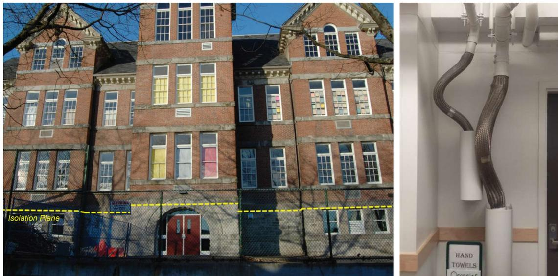
**Figure 1-3:** Strathcona Elementary column-top isolation scheme and flexible mechanical connections
