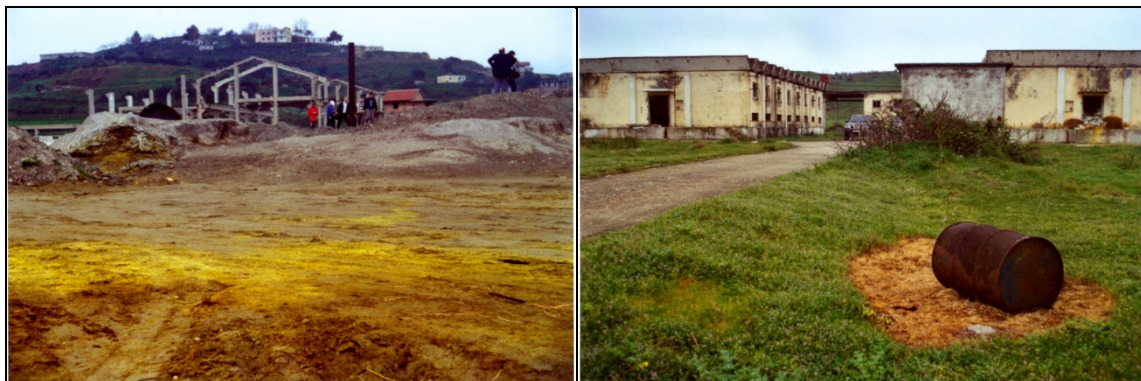
Figure 2.1 Chromium contamination at abandoned chemical factory in Durrës – Albania. At 2006, the area was contaminated with Lindane/ HCH and hexavalent chromium due to a former chemical plant [48]. Left, change on vegetation in same area due to soil contaminants. Reprinted from United Nations Environment Programme Disasters and conflicts[49]
