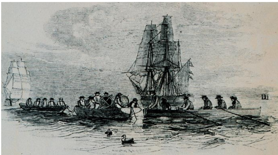
Figure 2.14. Artist's rendition of the crew of HMS Erebus measuring ocean depth using the 5000 fathom-long line created by Captain Ross (NOAA, 1840).
