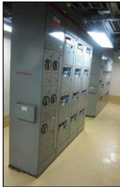
**Figure 2-5:** Motor control center (MCC) [32].
