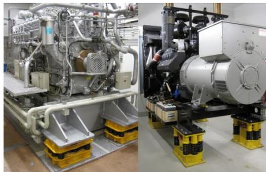
**Figure 1-3:** 3D isolation including spring and damper [6]
