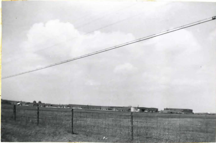
Photo 38. The R.C.A.F. Flying Station, west of Mount Hope. The hangers are in the right background, while the recreational buildings and living quarters are in the center and left foreground.
