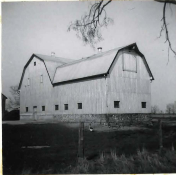
Photo 70. A good steel barn.
