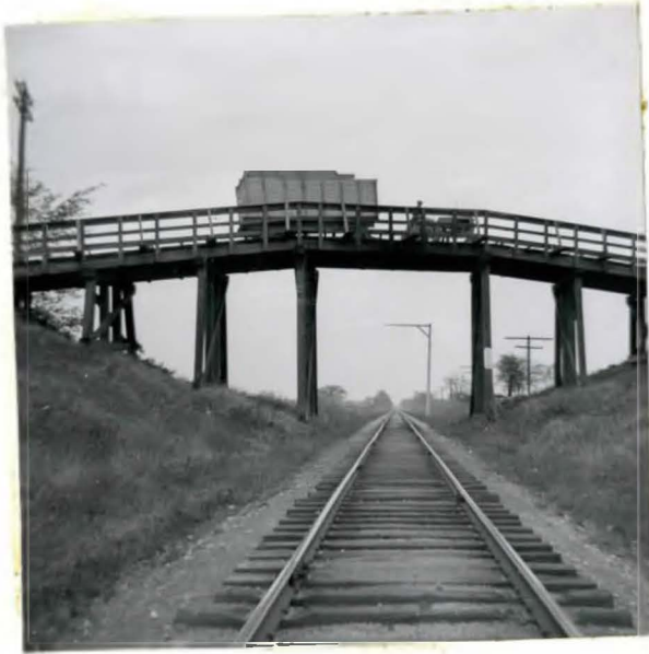
Photo 76. One of the narrow, steep and dangerous one-way wooden bridges crossing the Canadian National Railway through Glanford. A level crossing is recommended in place of the bridge.
