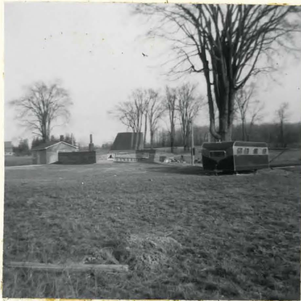
Photo 26. Fourth class housing. A cellar dweller. Three stages of development can be observed from this photograph. From trailer to cottage to cellar.
