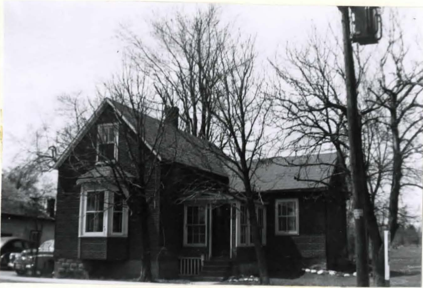
Photo 24. A well constructed old frame third class house, which has been covered with imitation brick.
