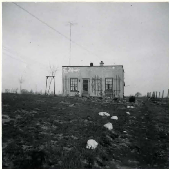
Photo 27. A fourth class, two room, cement block building, located along Highway No. 6. Note the T. V. aerial.
