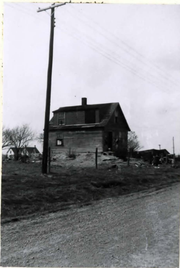
Photo 28. A fourth class, two story frame house. Note the litter in the yard. It is located south of Hannon.
