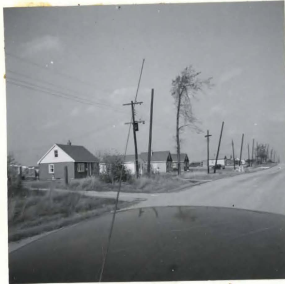
Photo 74. Ribbon development along County Road 33, south of Hammon. Houses are mainly fourth class. Without proper planning it could become a slum district.
