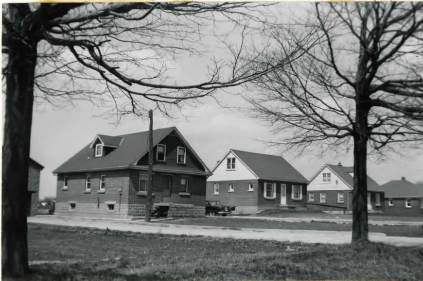
Photo 21. Second class houses north of Mount Hope along Highway No. 6. Well built brick, frame, or half brick, and half frame, of good size, well kept, and having the necessary conveniences, constitute this class.
