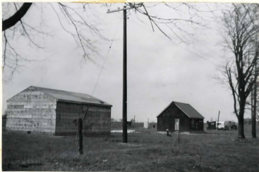
Photo 29. Fourth class housing south of Hannon. Three stages of development in owner built houses can be noted. From the trailer in the background to a plain wooden building to a tar papered building.
