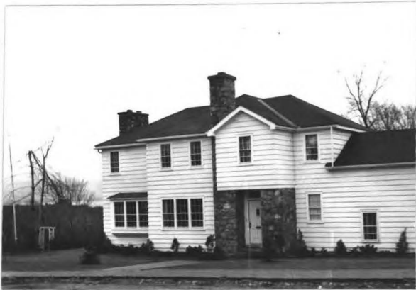
Examples of Class one housing in the Priest Hill area of North Bay.
