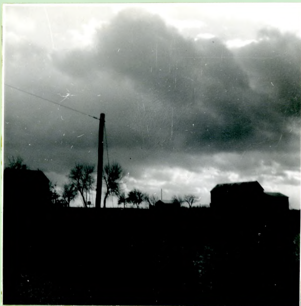
Fig. 47a. North Albion - Robinson farmstead in Sample Block #3. This is a 100 acre general farm. Note the typical size and shape of the house and buildings. A farmpond in the foreground illustrates how important they are becoming to the farm economy.
