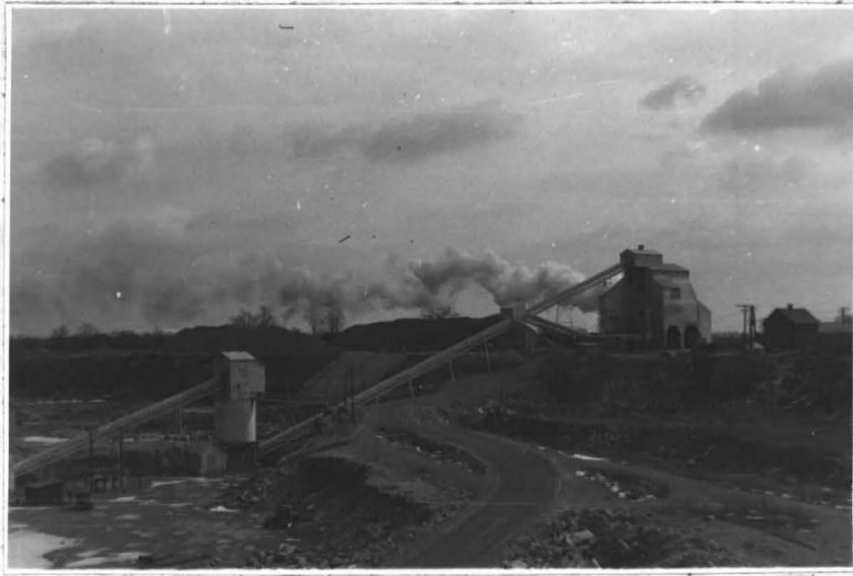
The Haldimand Quarries and Construction Co. Ltd., at Hagersville.
