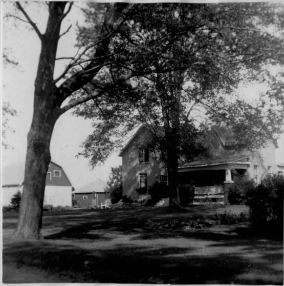
Fig. 5. A well-kept first class farmstead on the sand plain.
